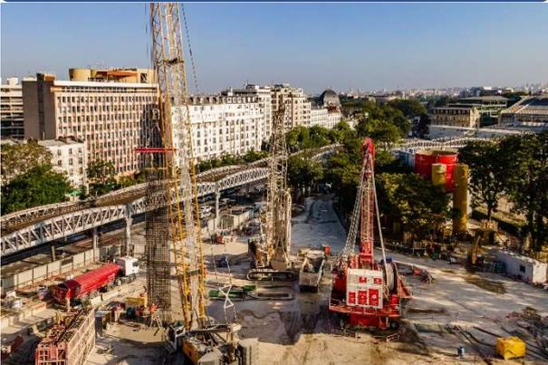
This water storage basin, of 50 metres in diameter and more than 30 metres deep, will store over 50,000 cubic metres of water. This project is an important investment of the Parisian city to control and manage the wastewater that currently is discharged into the Seine.
